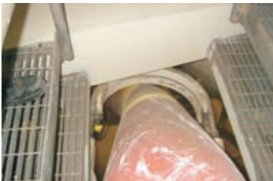
▲ Assembly of pipe whip restraint is not compliant with installation specification
