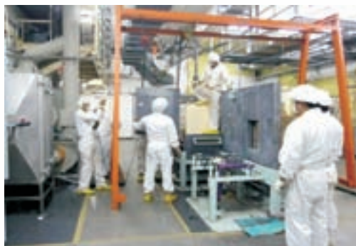
▲ Dismantling of Lead Shielding Blocks
