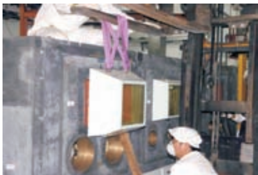
▲ Dismantling of Analytical Lead-cell Line
