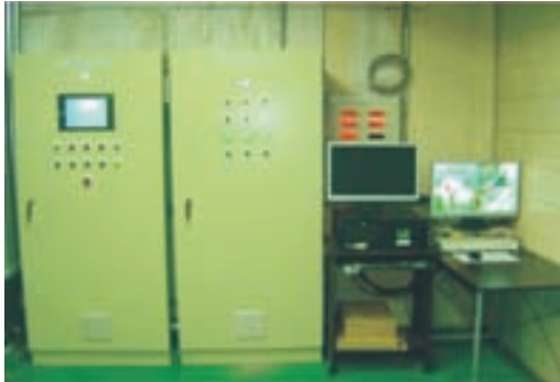
▲ Programmable logic control system and monitoring system
