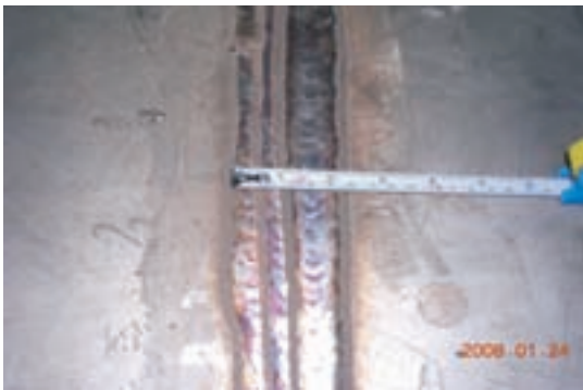
▲ Root opening of weld joints are not accepted when assembling the liner of the suppression pool
