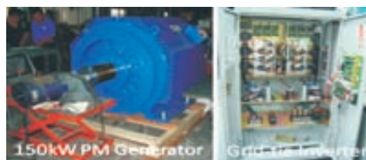
▲ The 150 kW PM generator and the grid-tie inverter
