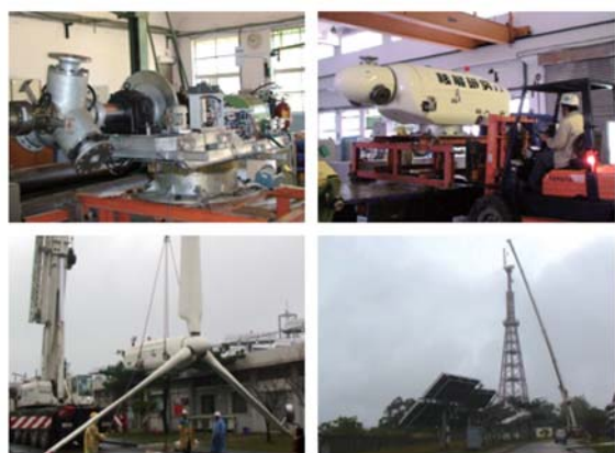
▲ Assembly and Installation of Wind Turbine
