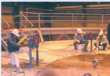
▲ Drilling Samples on Top of Biological Shielding
