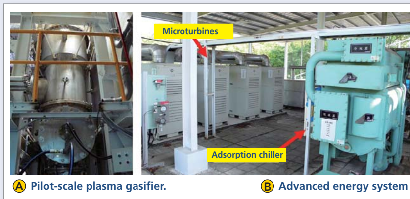
▲ A Pilot-scale Plasma Gasification Plant for Bio-electricity Generation.
