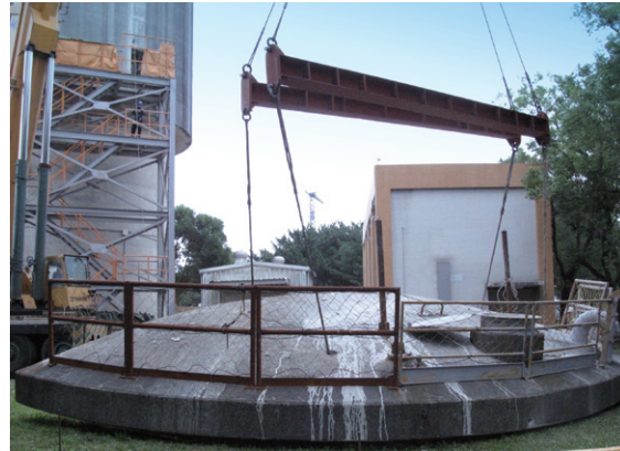
▲ Concrete Block Lifting Operation
