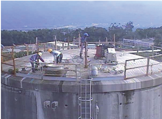
▲ Top Cover Cutting Operation
