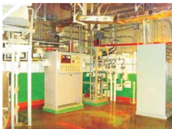
Post-Accident hydrogen Monitor in RAB
