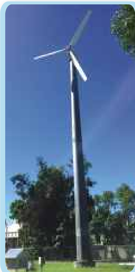
Fig. INER 25kW horizontal axis wind turbine and support structure
