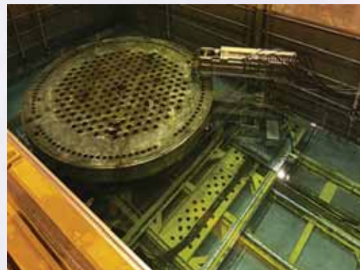
Underwater cutting of high-dose-rate components
