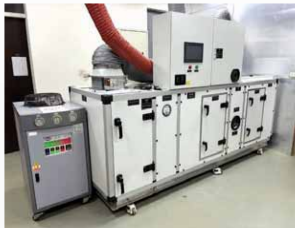
Dryer of adsorption rotary wheel
