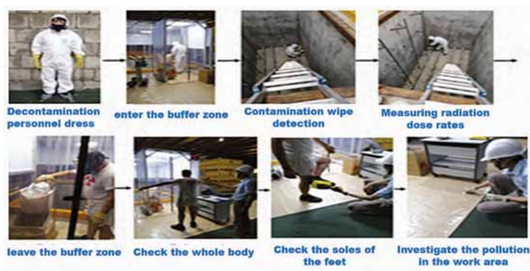
Fig.1. On-site decontamination work
