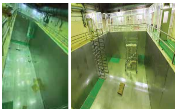
Fig.5. The additional stainless steel isolation plate in the fuel pool
