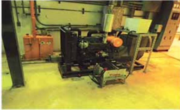
Fig.3. Equipment related to backup power of the HIS system in Kuosheng NPP
