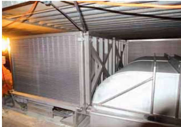
Fig.4. Strainer Onsite Installation
