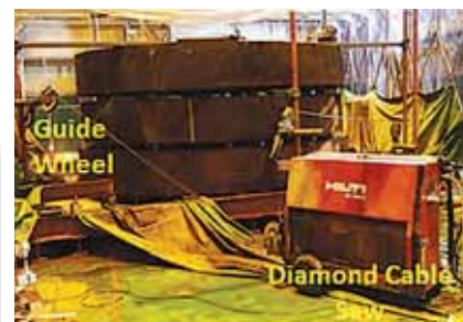
Fig.4. Upper biological shield cutting operation
