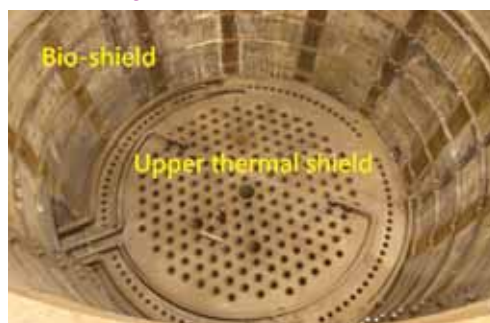
Fig.3. The thermal shield through the tube on TRR
