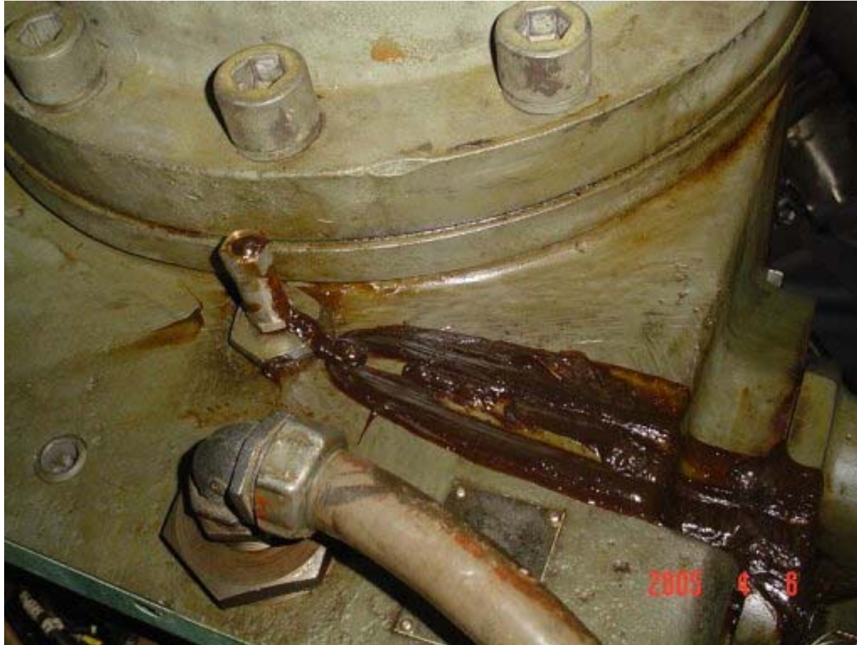
Discharge from Limitorque Grease Relief Valve - Evidence of elevated main gearbox temperature
