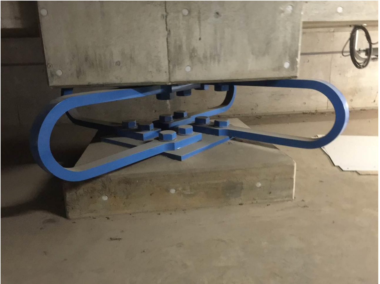
圖 31 僅 U-shape steel damper
