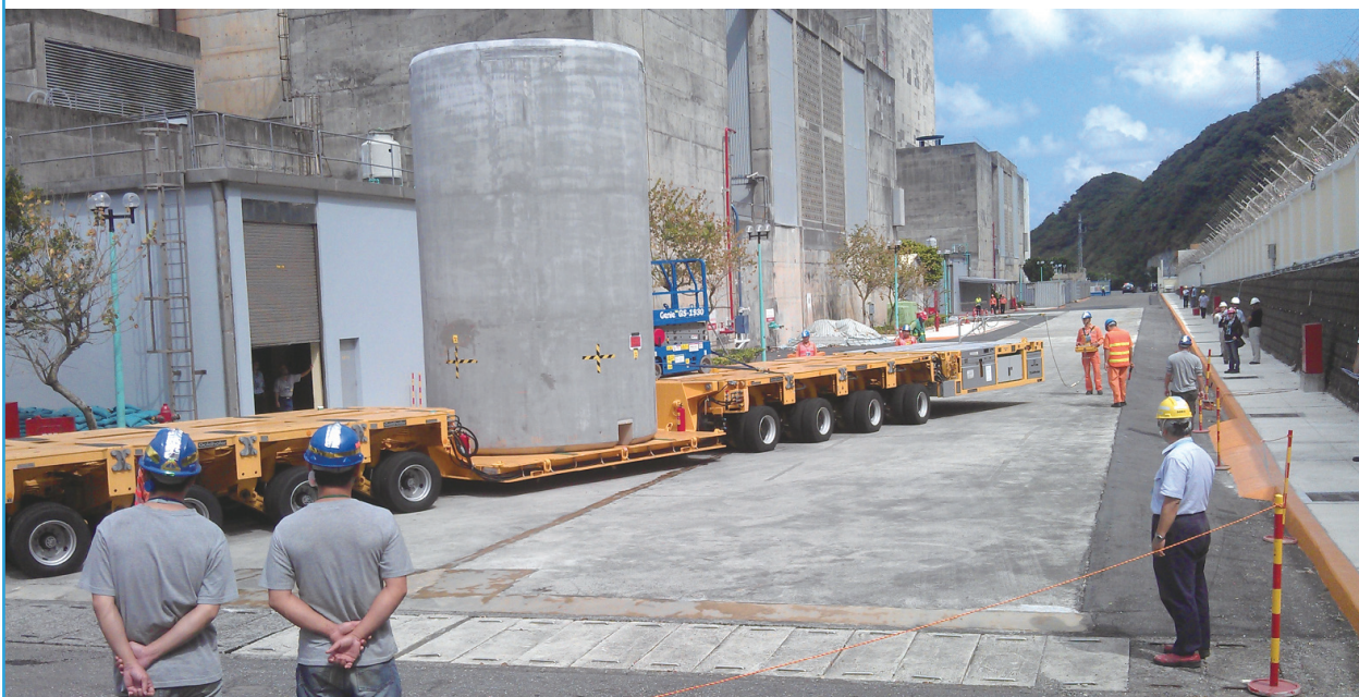
▼ Fig.7 Concrete Cask Movement using Dolly Inside Chinshan NPP.
