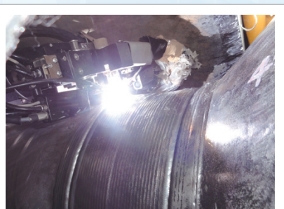
▲ Fig.3 WOL on the feedwater nozzle of Kuosheng Nuclear Power Plant Unit 1.
