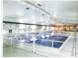
The underground part of Clab consists of two rock caverns. Each rock cavern contains four water pools for storage plus a reserve pool. All handling underground is performed by a handling machine. When a storage canister comes down, the machine is used to lift it out of the elevator cage. The machine then places the storage canister in a predetermined location in one of the pools.
